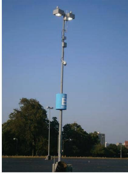
*HD video cameras mounted on the outside of the structure serve two purposes: the higher camera provides views of parking areas; the lower cameras view the sidewalks and gate entrances. In parking lots, of which U.S. Cellular Field has six, wireless technology transmits images to the VMS.*
